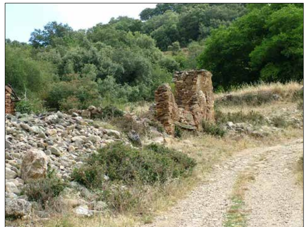
Figure 17. Another example of a construction abandoned in a recent era. The photograph was taken in La Balouta (Leon, Spain).
